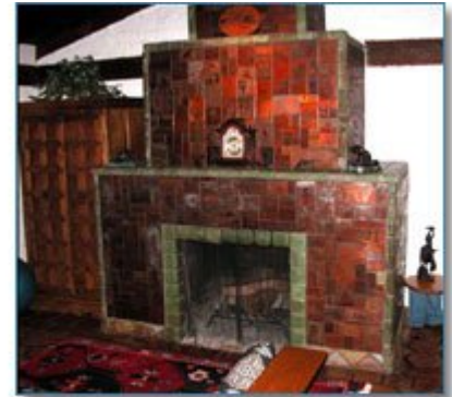
The family room fireplace is covered in copper printing plates that look like iridescent tiles.
