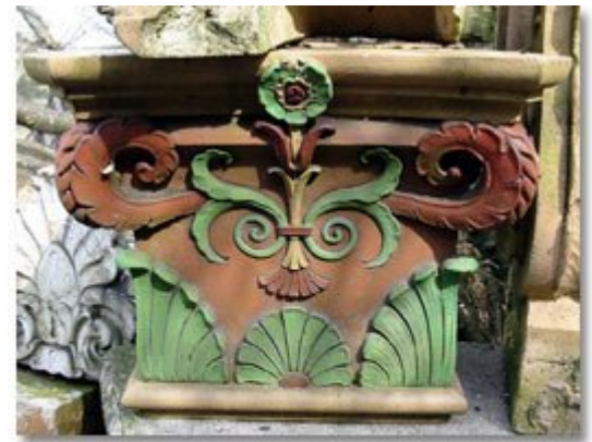
Architectural terra cotta from Park Point Elementary School, one of many "Orphans" on display at the Fairlawn Mansion.
