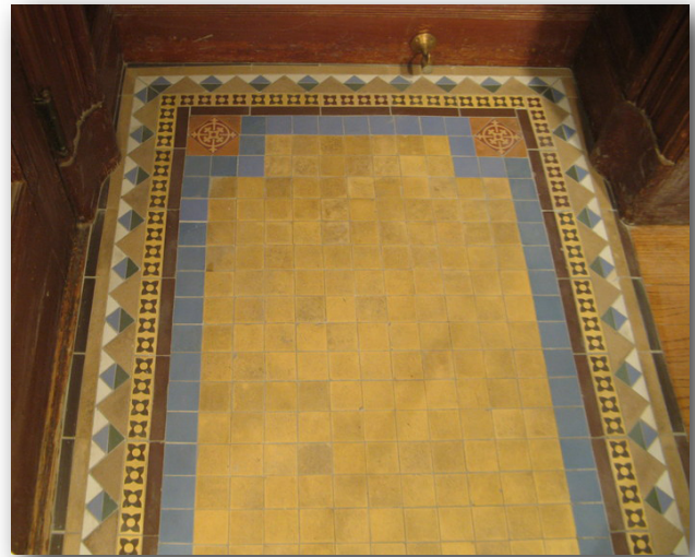
The completed geometric/encaustic tile floor at Ravenswood.
