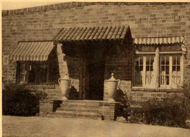
Main Entrance to Offices
