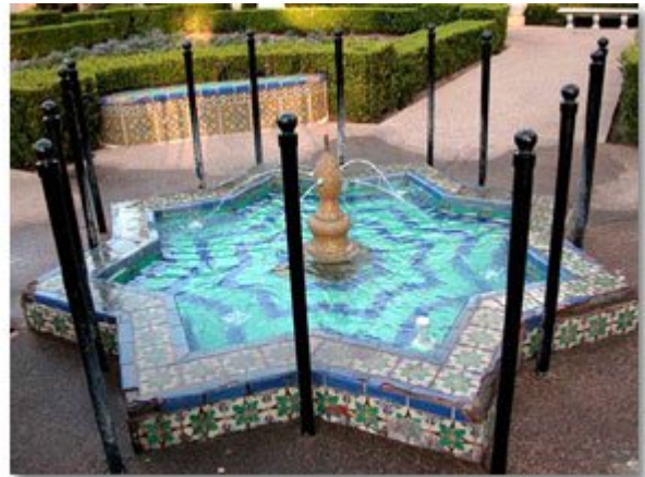
Central fountain in the Alcazar Garden. Note the damage to the tilework from skateboarders and the barrier posts recently installed to minimize further harm.
