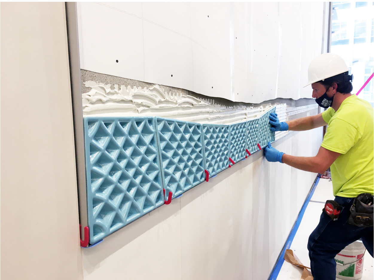
Installing (direct set) by Artisan Tile & Marble Co of NJ, Inc
