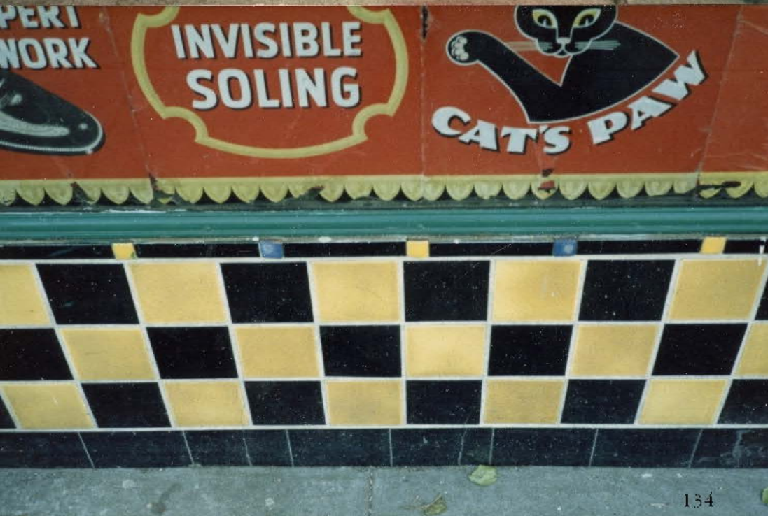
134. San Pablo Ave. & Dwight, Berkeley (This section has been painted over, seems intact underneath)
