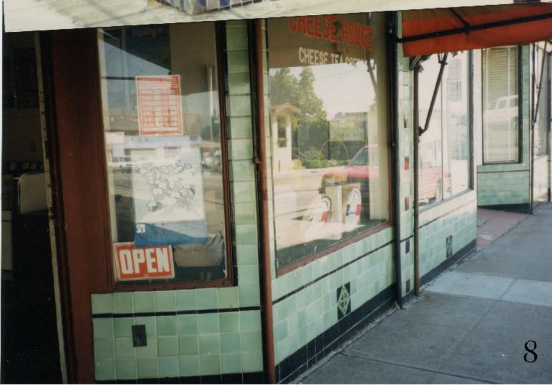
8. 3046 MacArthur Blvd., Oakland (still intact 3/5/17)
