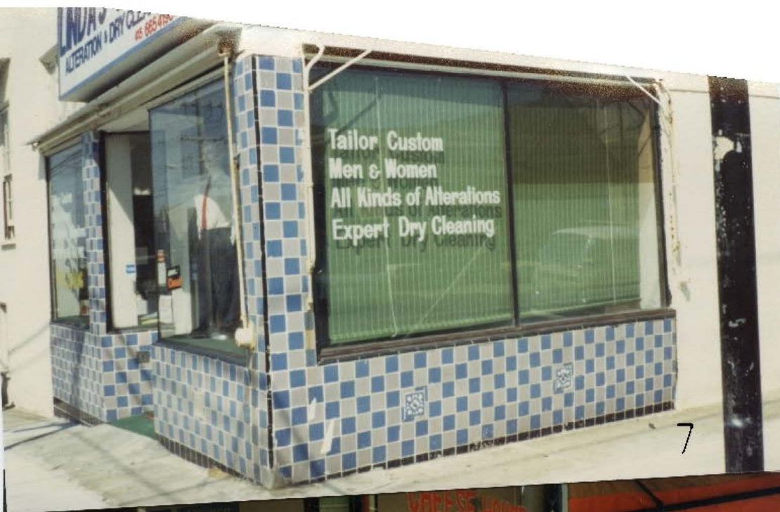
7. 1498 9 th Ave., S.F. (tiles have been removed – plain stucco 3/3/17)
