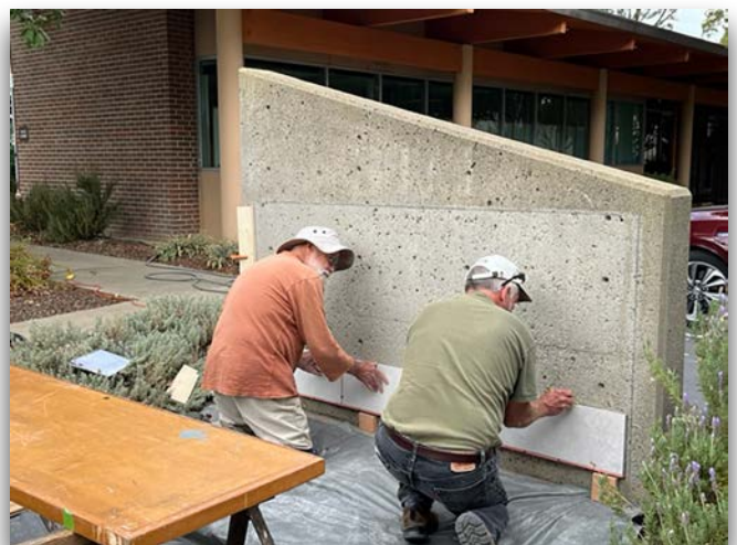
Setting the first row, note support blocks.
