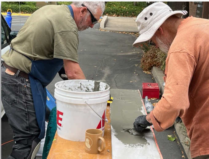
Kenyon (left) and Shelby back buttering the first layer.
