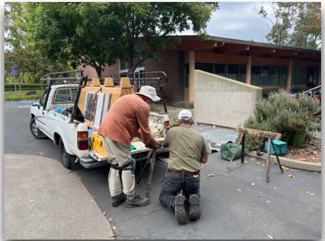
Unloading the components from the A frame.
