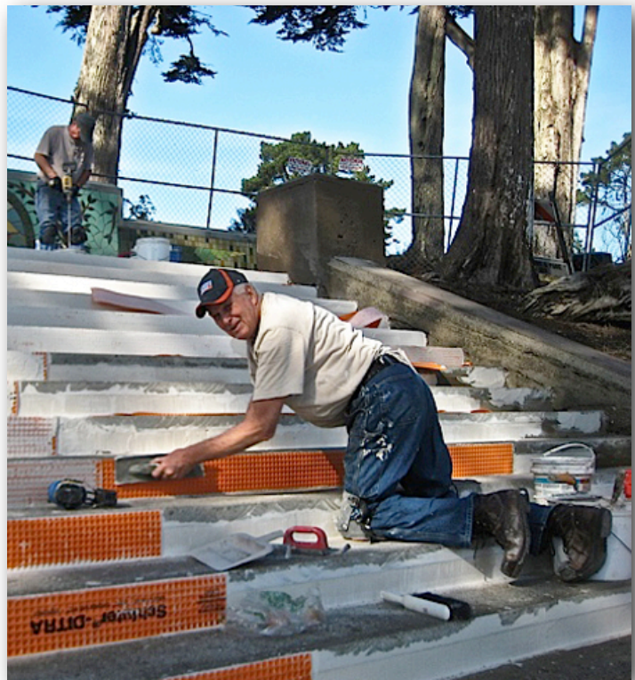
Riley Doty installing Schluter Ditra matting.
