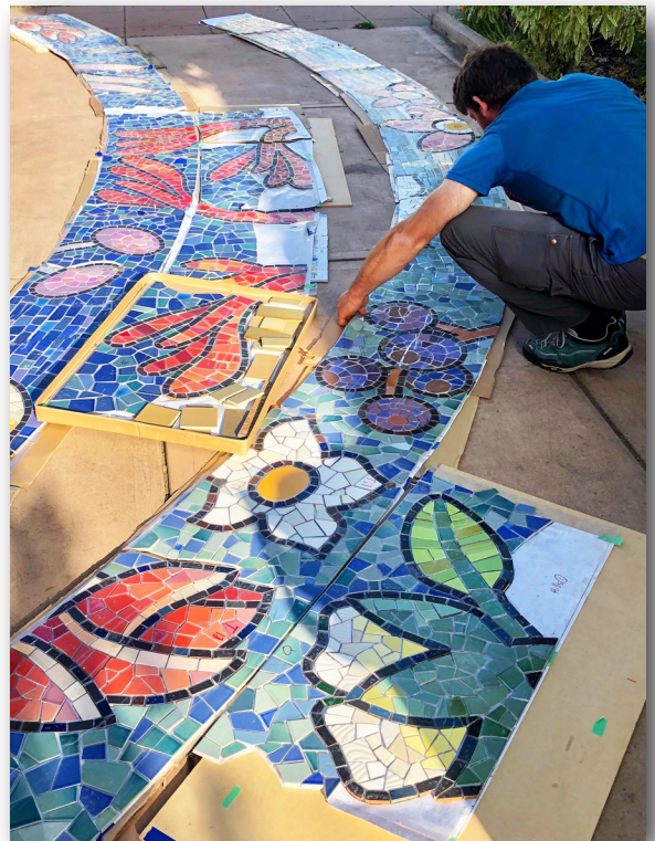
Lofting the mosaic prior to installation.
