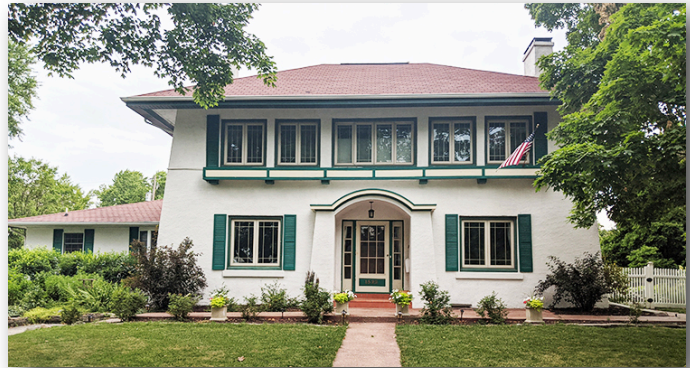
The Finley's prairie style home in Bloomington, Illinois, designed by architect Arthur L. Pillsbury in 1910.
