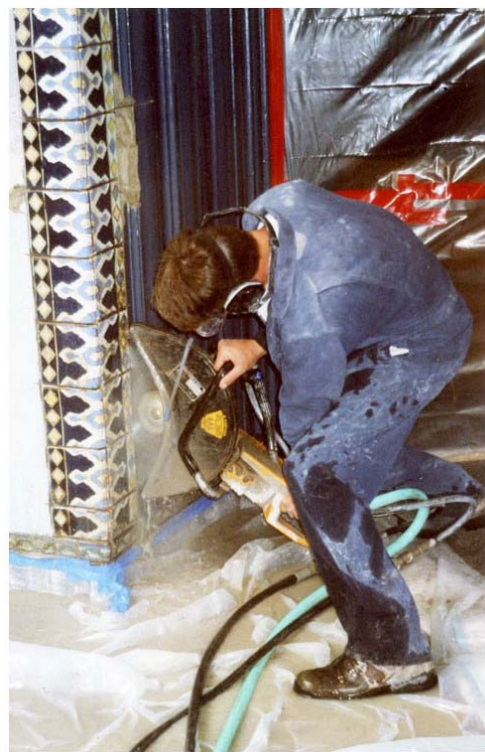
James Dawes carefully cuts into the grout joint, removing the historic Solon & Schemmel tiles from the old Steinhart Aquarium. Photo courtesy of Riley Doty.
