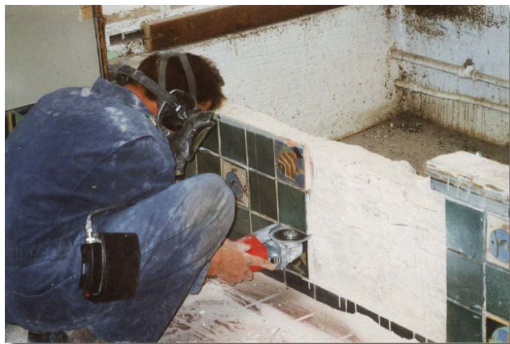
Protected by the “rebreather,” James Dawes demonstrates the extraordinary skill needed when removing old tiles. Photo courtesy of Riley Doty.
